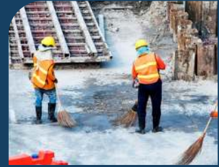
Building Restoration services
